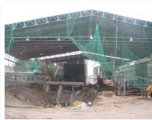
over a period of several months about water seepage and cracks forming in the basement walls of the archives storage stronghold. In fact, damages of this kind had been noted for the past several years along the same street as work on the subway tunnel progressed. A medieval church bell tower had to be propped up in 2007 because it began to lean by several degrees. A month before the collapse, the archives building had sagged towards one side showing cracks in
