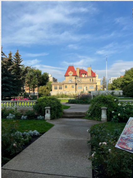
Site visits in Calgary, 2022: Lougheed House
